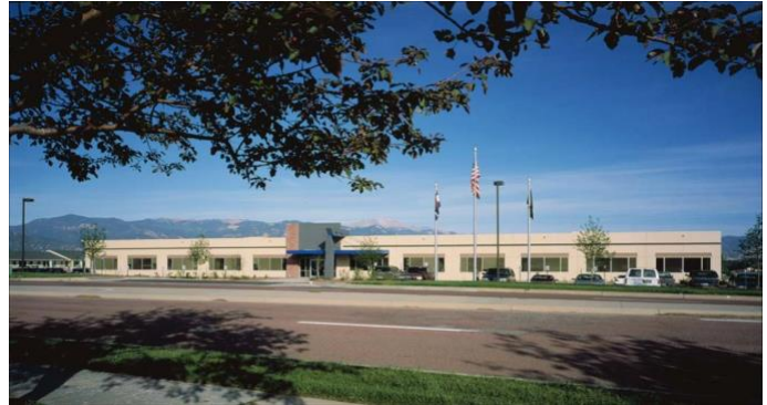
MITRE Corporation build-to-suit, Colorado Springs, CO
